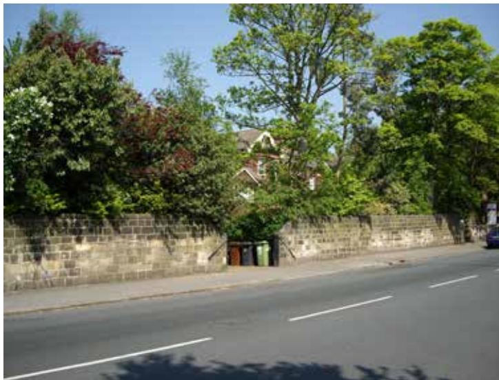
Fig. 3.18 Original stone wall in Harrogate Road
