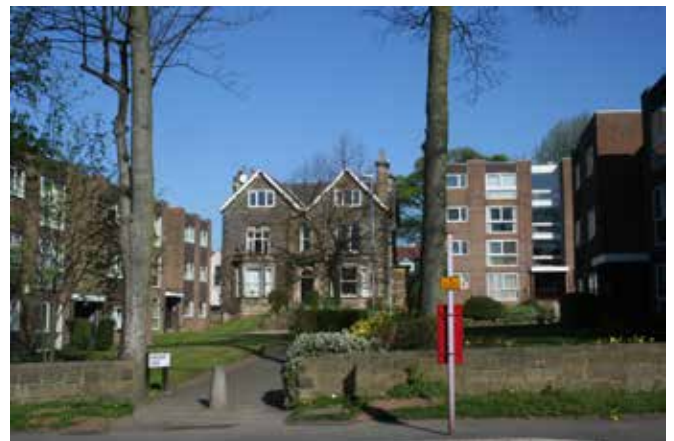
Fig. 3.95 Modern apartment blocks (Kingsway Ct) surrounding Keldholm, a substantial Victorian house
