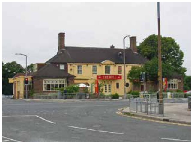
Fig. 2.16 Chained Bull public house (now demolished)
