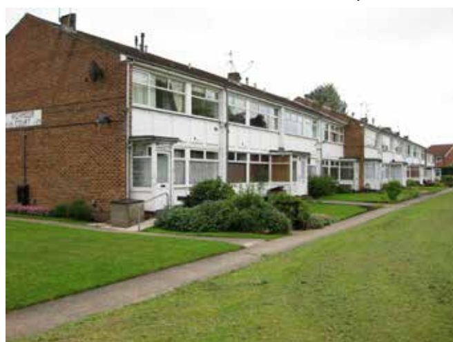
Fig. 3.60 High Moor Court to residential accommodation may be suitable here in future and the parade would benefit from landscaping.
