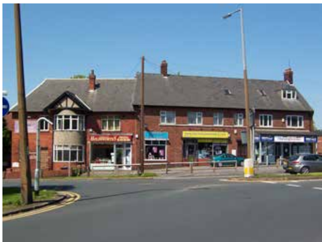
Fig. 6.5 Shops at northern part of Harrogate Rd
