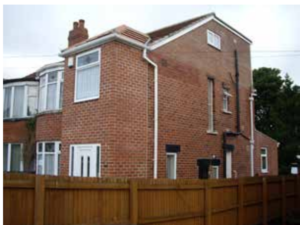
Fig. 3.20 Extension markedly changing original roof line
