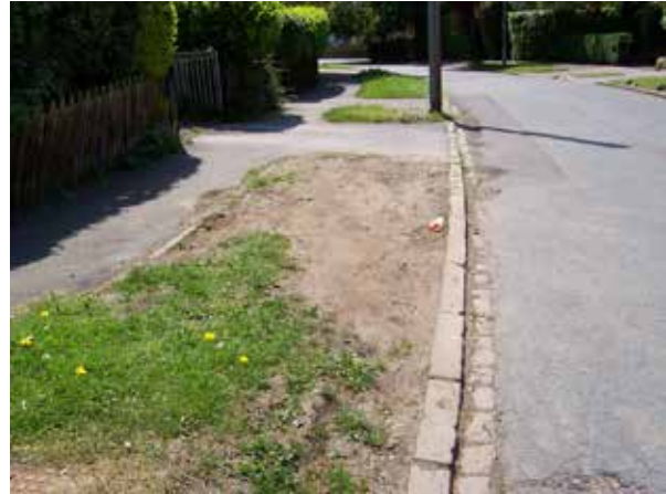
Fig. 3.25 Grass verge damaged by parking
