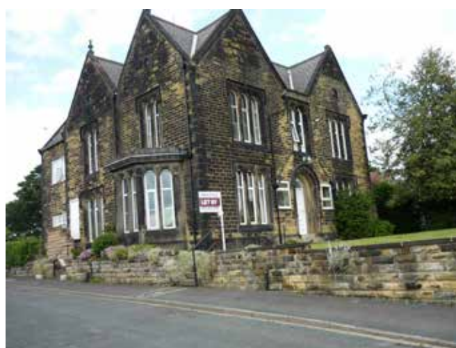
Fig. 3.84 Victorian villa in Allerton Grange Walk
