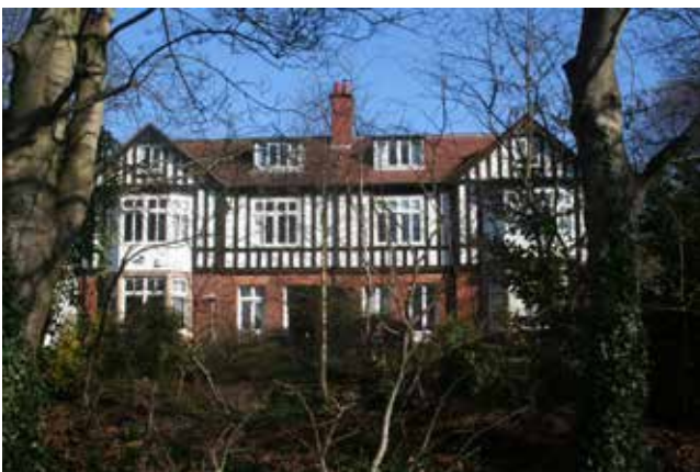
Fig. 3.40 Substantial early 20thC semis in Sand Hill Lane
