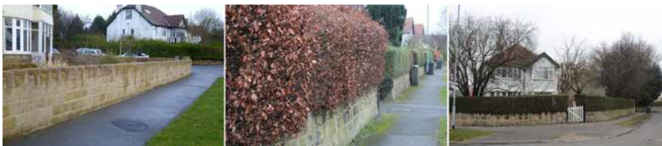
Fig. 3.16 Stone boundary walls
