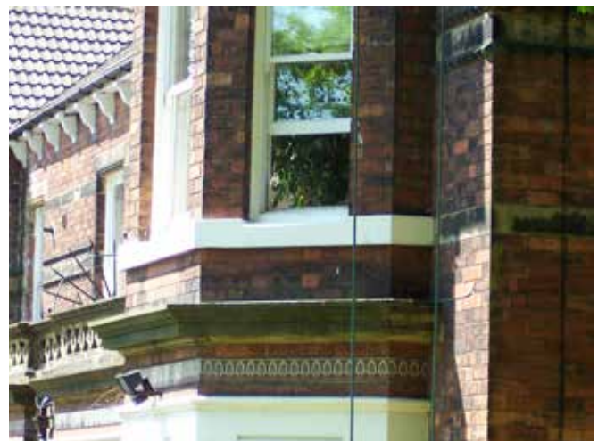
Fig. 3.101 Architectural detail at 305-307 Harrogate Rd
