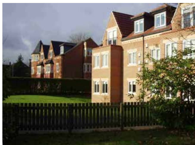
Fig. 3.52 Lime Tree Lodge and Parkway Lodge
