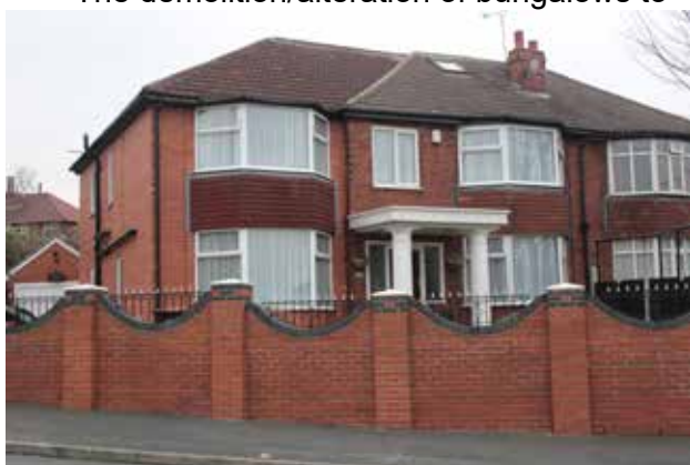
Fig. 3.22 Extension with portico out of keeping with original building
