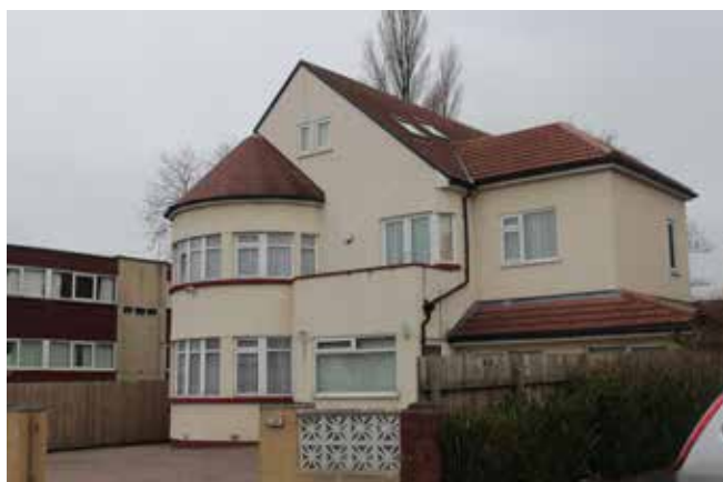
Fig. 3.23 Extension which overwhelms the original flat-roofed art deco building
