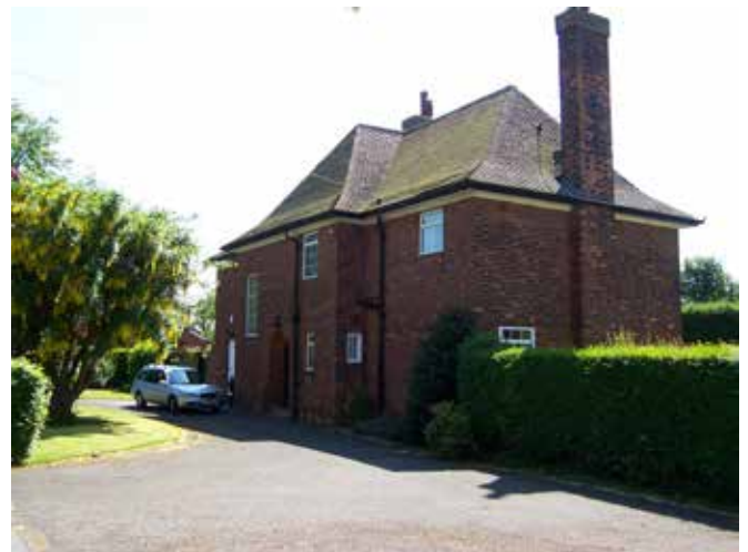
Fig. 3.93 Substantial detached house in Moorland Dr.
