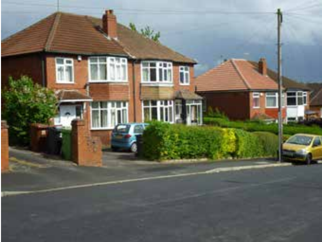
Fig. 3.66 Semi-detached houses in Moor Allertons
