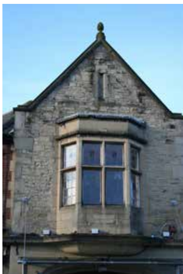
Fig. 3.36 Mock oriel window on stone face of Corner House
