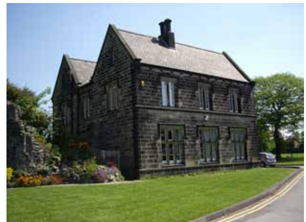
Fig. 3.80 Roman Catholic presbytery adding greatly to the pleasant character of the area.
