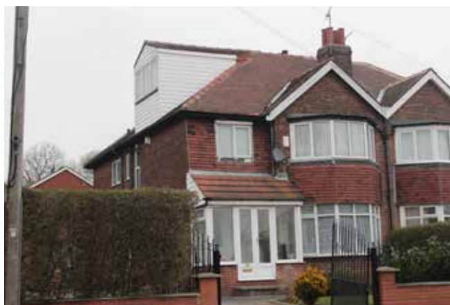
Fig. 3.21 Extension finished in unsympathetic materials
