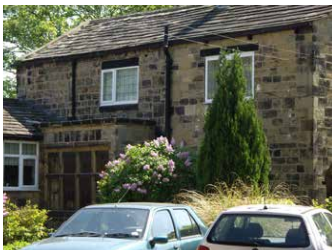
Fig. 3.82 Stone cottages behind 284 Harrogate Rd
