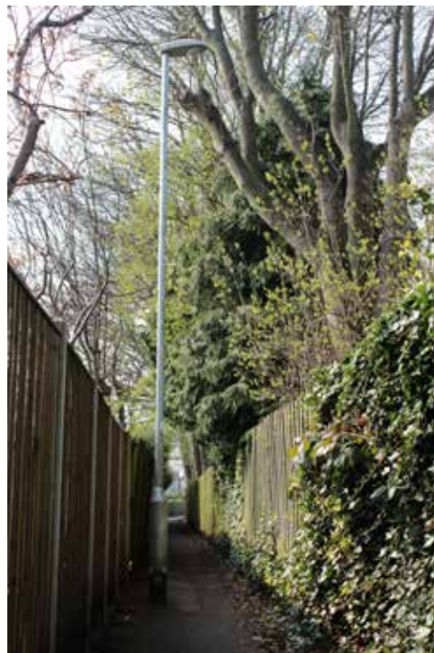
Fig. 5.13 Lamppost obstructing footpath (now repositioned)
