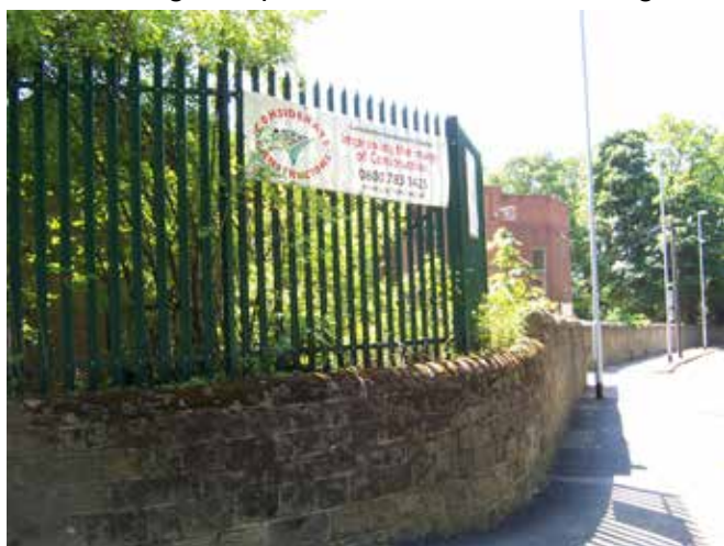
Fig. 3.57 Original boundary wall at Donisthorpe Hall
