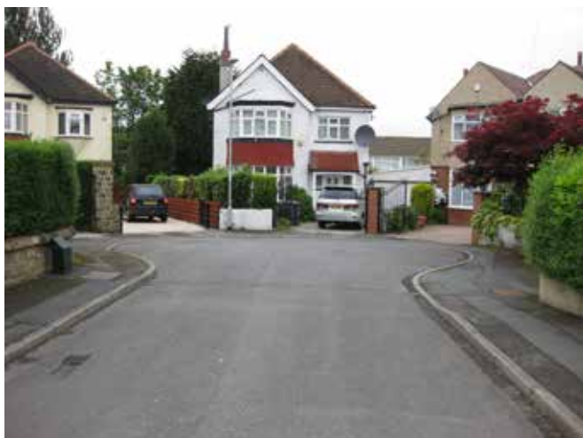
Fig. 3.48 Detached house in Southfield Dr.
