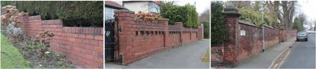
Fig. 3.17 Brick boundary walls
