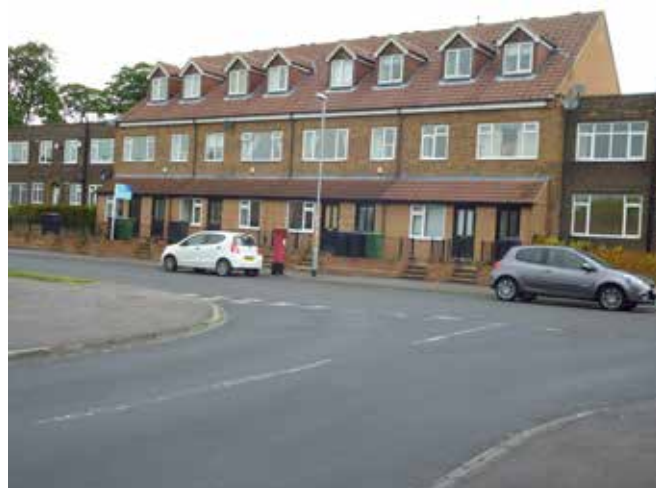
Fig. 6.7 Shops converted to houses in High Moor Cres
