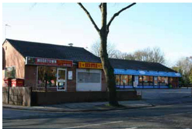
Fig. 6.8 Fast food outlets and fish restaurant in Street La
