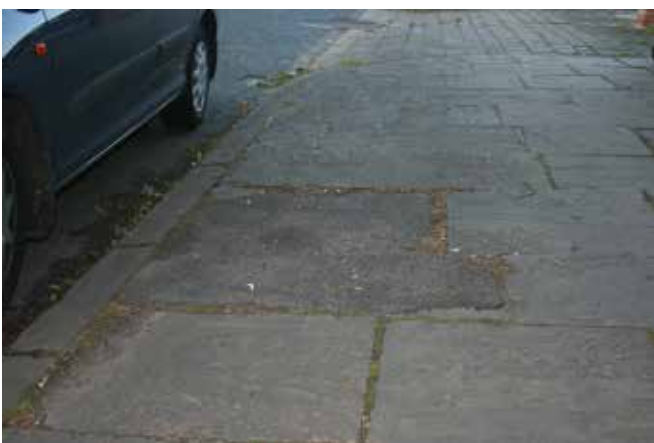
Fig. 4.9 Tarmac replacing felled tree in Street Lane
