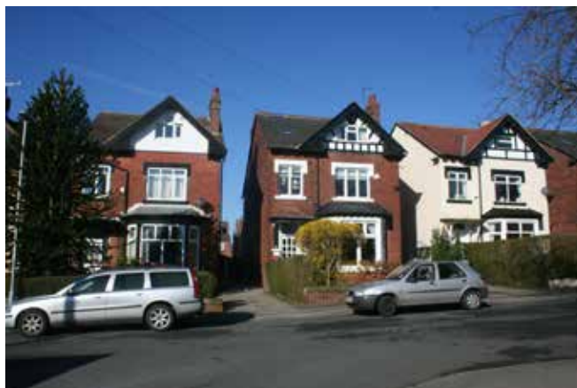
Fig. 3.65 Detached houses in Bentcliffe La
